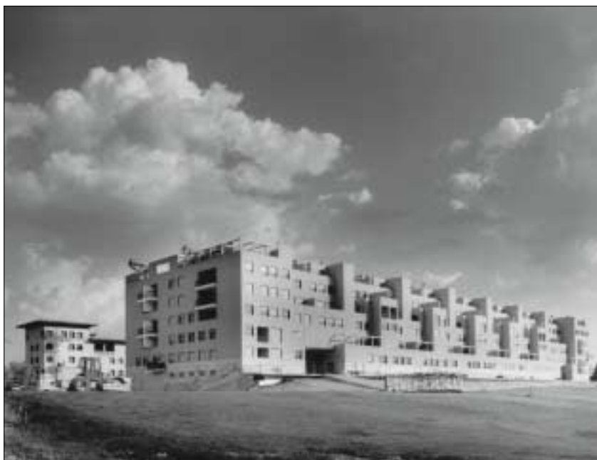
Some of the buildings built by Pirelli & C. Real Estate in the Bicocca area in Milan.
